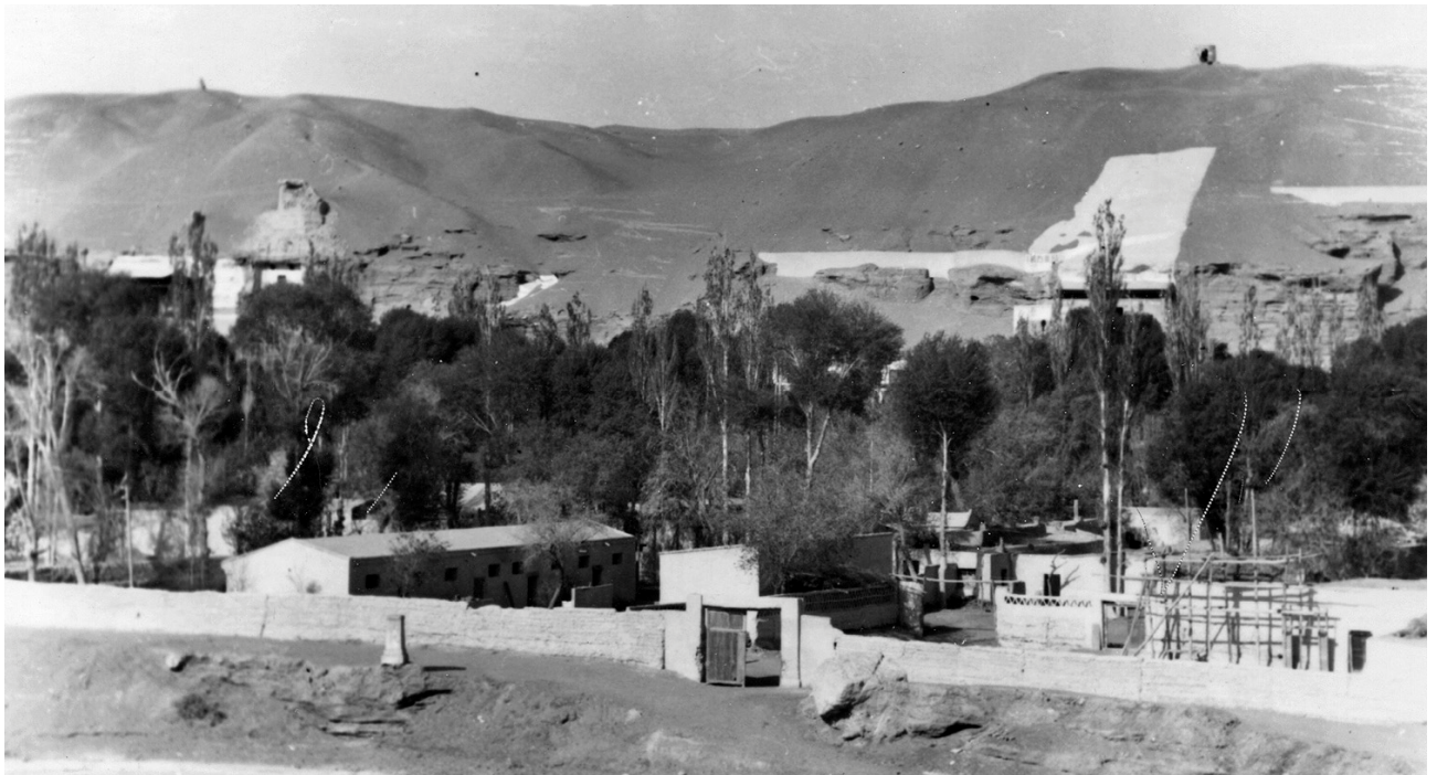
Figure 10: A protective wall built around the Mogao Caves in the 1940s by the National Dunhuang Art Institute.
