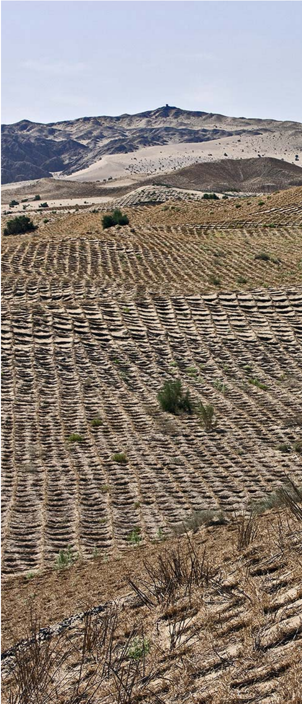
Figure 23: The “checkerboard” barriers to obstruct sand.
