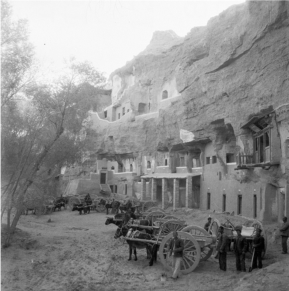
Figure 7: In the 1950s, the Dunhuang Institute for Cultural Relics clears the sand accumulated in the cave area.
