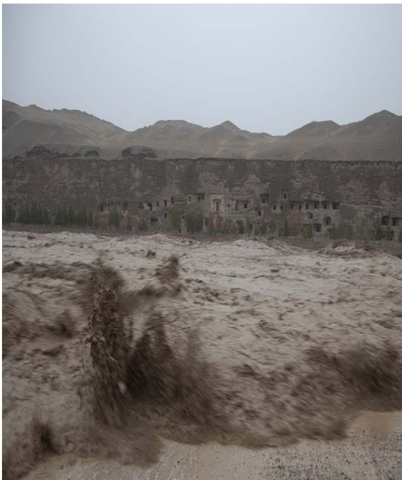
Figure 21: On June 6, 2011, a torrential rainstorm hit the Mogao Caves
