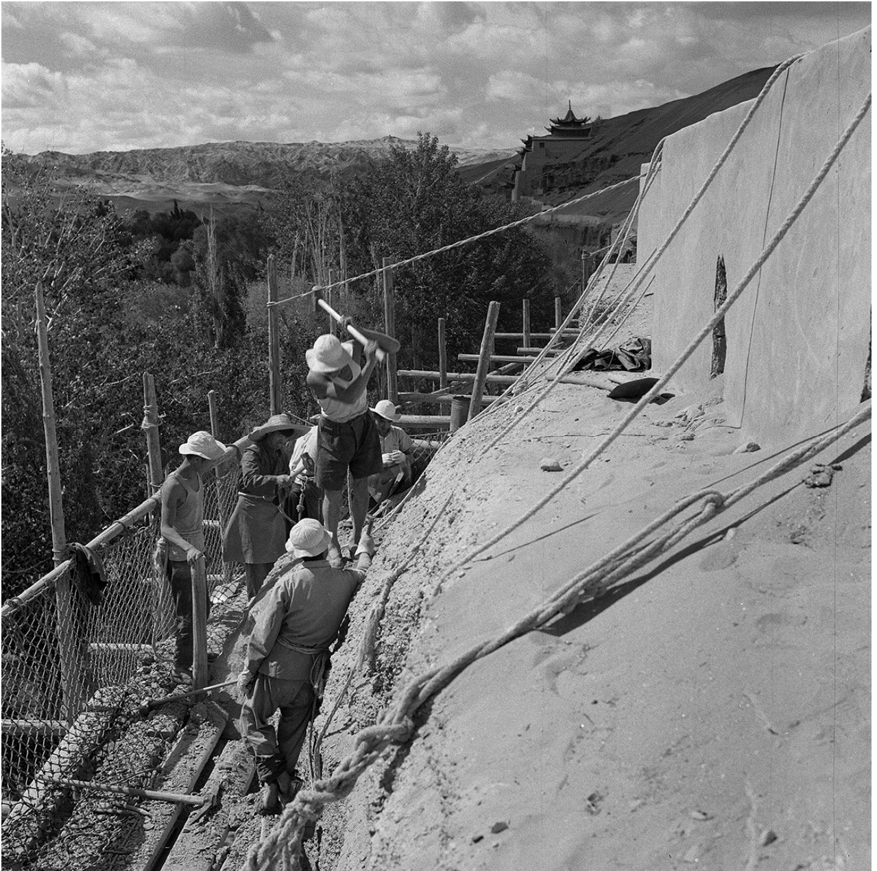
Figure 18: Stabilization of rock body and clearing of pumice stones at the top of the cave in July 1965.
