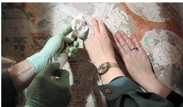
Figure 22: Grouting of the wall paintings
