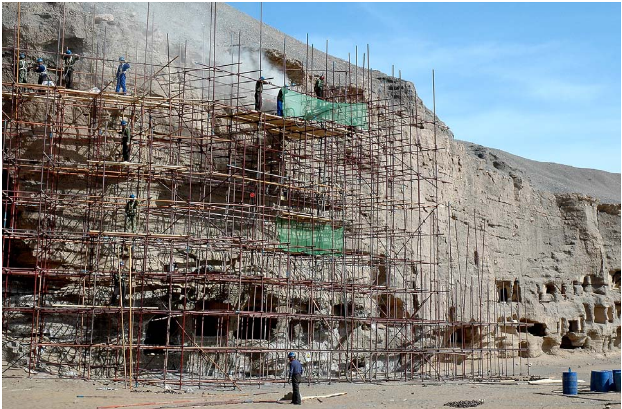
Figure 20: Stabilization work at the northern cave area in 2004.
